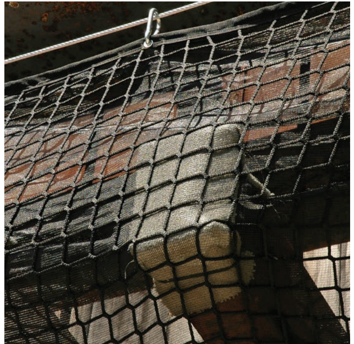
Dual layer protection to contain fine particles.
