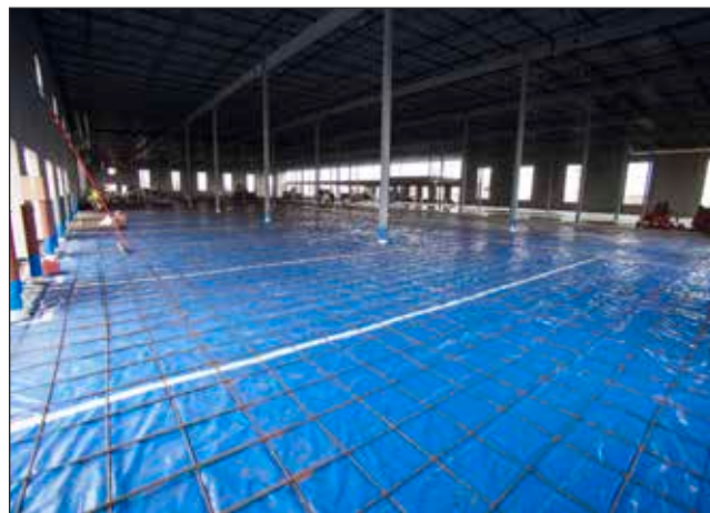
Vapor Barrier - Commercial
