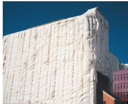
Reinforced polyethylene tarps protect crews and materials in hard weather conditions.
