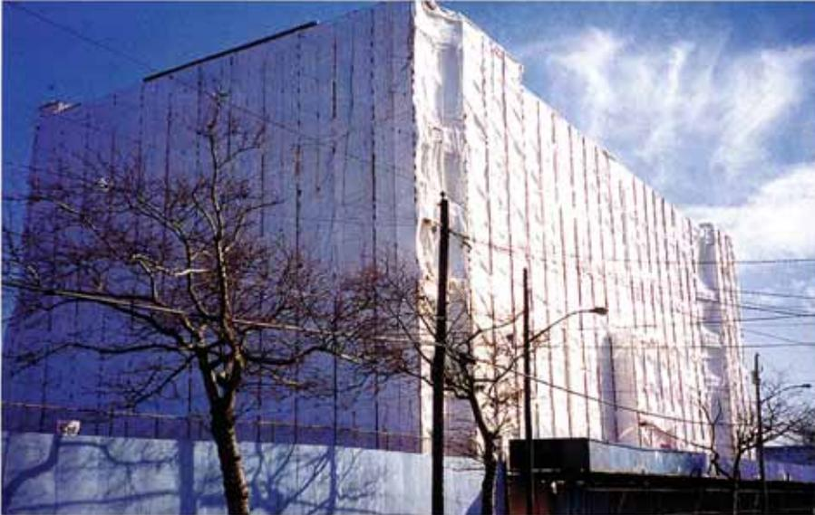
Weather enclosures protect construction crews from wind chill and precipitation, allowing them to comfortably work in a heated environment through even the most inclement weather
