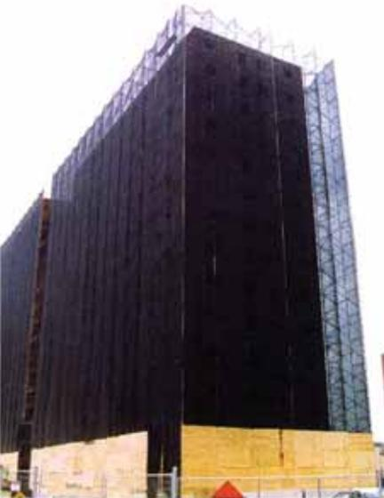
Mesh netting prevents sand, dust and other construction debris from becoming a safety hazard, while providing constant air circulation and high visibility for work crews
